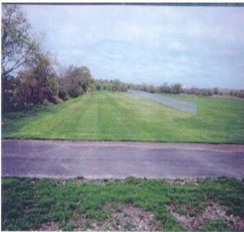
Middletown soccer field parking lot shortly after construction.
