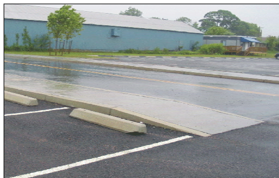
Porous asphalt parking lot at University of Rhode Island.
