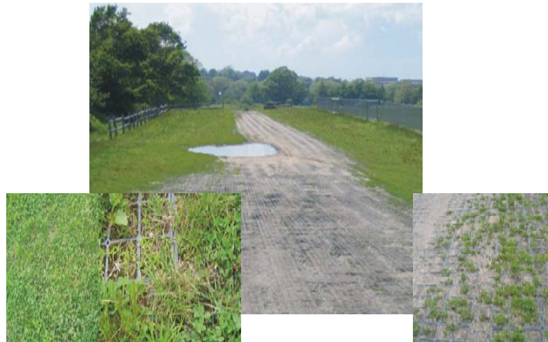
Middletown soccer field parking lot in June 2004.
