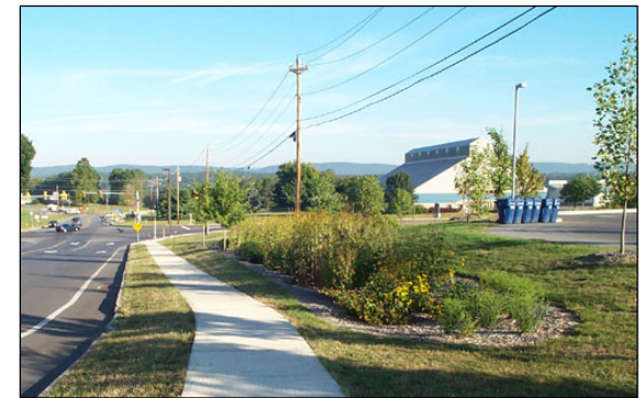
Porous concrete sidewalk at Penn State University (Source of photograph: Cahill Associates)
