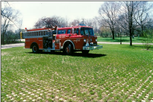
Fire access paved with Hastings Checker Block
