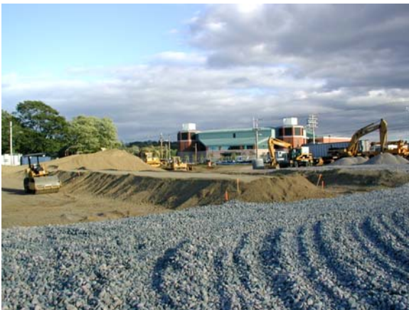
Soil excavation and placement of crushed rock.
