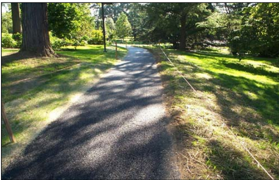
Porous asphalt pathway at Swarthmore College. (Source of photograph: Cahill Associates)
