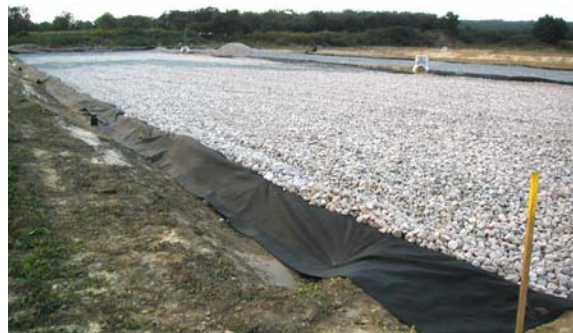
Stone reservoir surrounded by geotextile filter fabric.
